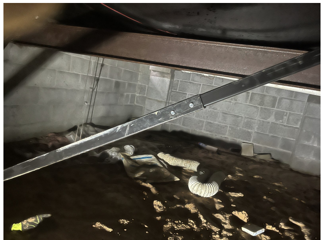
Adjustable side brace — keeps the home from shifting side-to-side.
