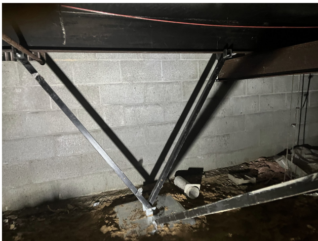
The brace ties into a solid anchor pad set into the ground below.
